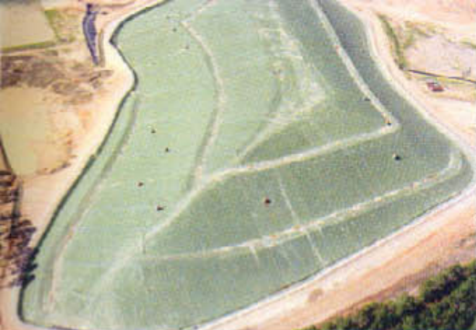
Photo 5 | An aerial view of a completed exposed geomembrane cover on a landfill in Florida. Pipe vents were installed for wind protection.
